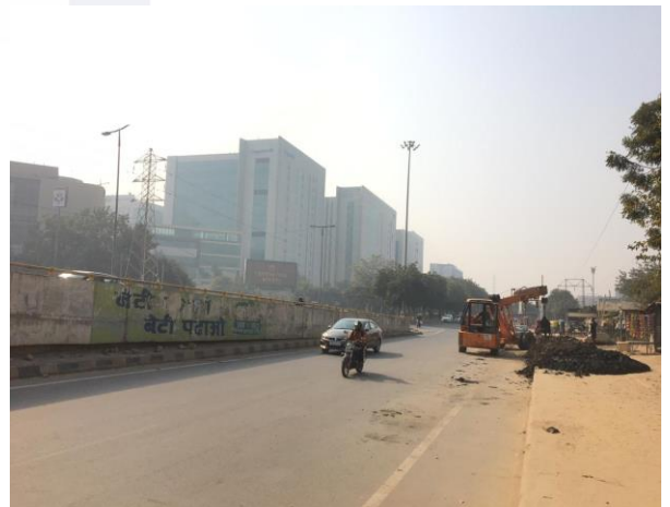
View of the Access Road
