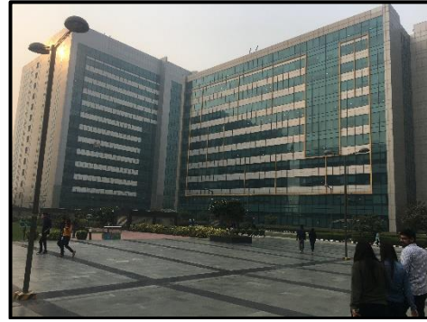
View of Tower 2 & 3
