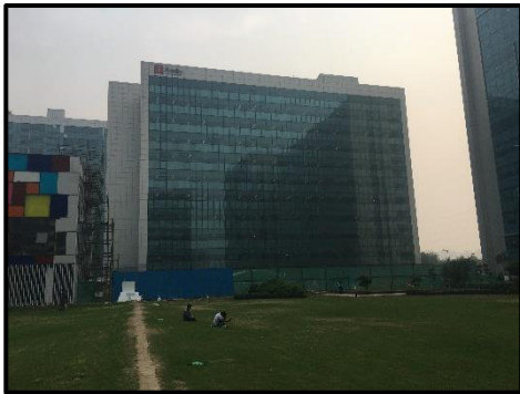
View of Tower 9
